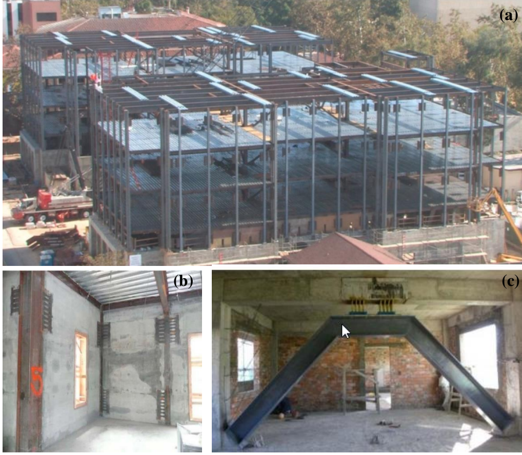
Fig. 2: Several structural applications of butterfly-shaped fuses[30]
